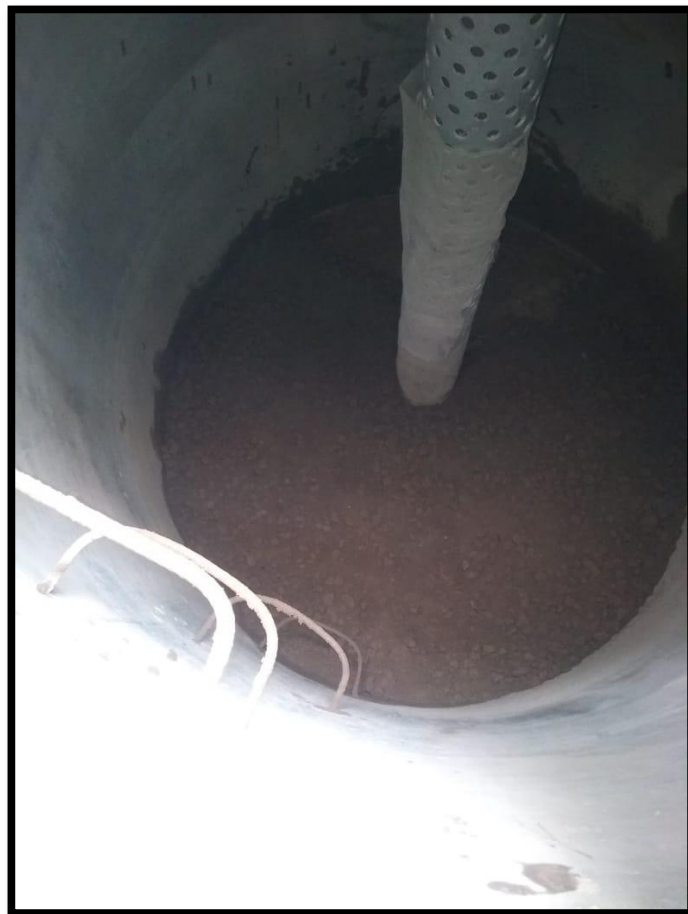
PIT AFTER CLEANING
